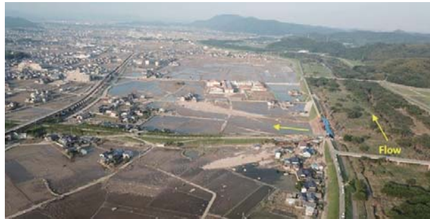
Flood damage in Mabi Town due to a levee breach along the Oda River
